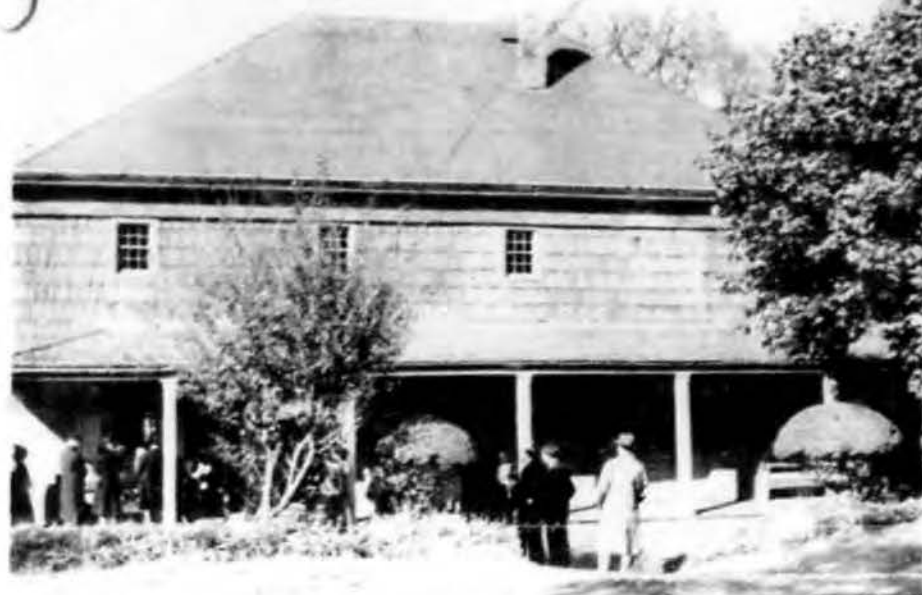
Friends Meeting House, Flushing, N. Y., built 1694
